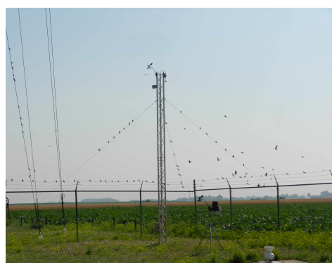
the small air inlet mast (6 m)
